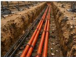
DUCTING INSTALLATION Installation of HDPE ducts for power, telecom and fiber optic cables.
