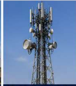
TELECOM TOWER INSTALLATION Installation of telecom towers with antennas and microwave dishes.
