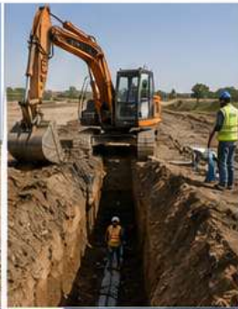
02 EXCAVATION WORKS Excavation for foundations, trenches and utility ducts as per design.
