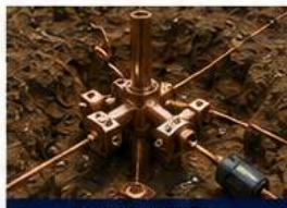
EARTHING SYSTEM Earthing system installation for equipment and lightning protection.
