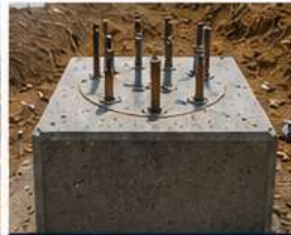
FOUNDATION COMPLETION Completed foundation with anchor bolts ready for tower erection.
