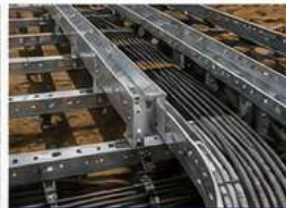
CABLE TRAY INSTALLATION Cable tray installation and route management at site.
