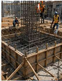
03 FOUNDATION WORKS Reinforcement, formwork and concrete works for tower and equipment foundations.
