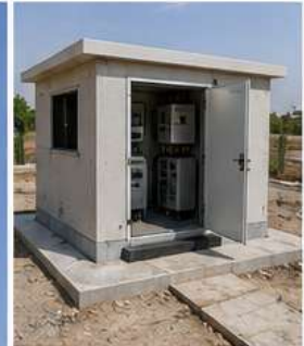
10 EQUIPMENT SHELTER SETUP Construction and installation of equipment shelters and outdoor cabinets.
