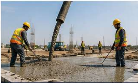
5. CONCRETE WORKS RCC structures, columns, beams, slabs and shear walls with quality concreting.
