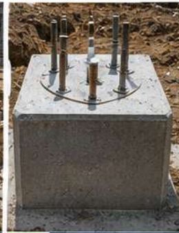
04 FOUNDATION COMPLETION Completed foundation with anchor bolts and curing for strength and durability.
