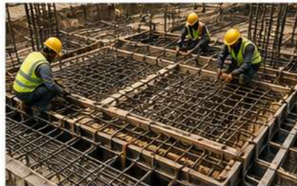
3. REINFORCEMENT WORKS Cutting, bending and fixing steel reinforcement as per structural drawings.
