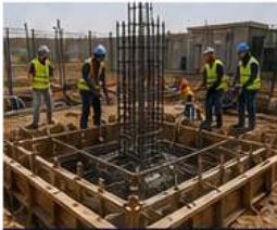
TOWER FOUNDATION WORKS Excavation and reinforced concrete foundation for telecom towers.
