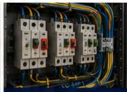
SURGE PROTECTION Surge protection devices for equipment and power lines.
