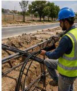
06 CABLE PULLING Pulling of power, telecom and fiber cables through ducts and conduits.
