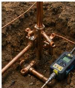
12 EARTHING & LIGHTNING PROTECTION Earthing system installation and lightning protection for safety and reliability.
