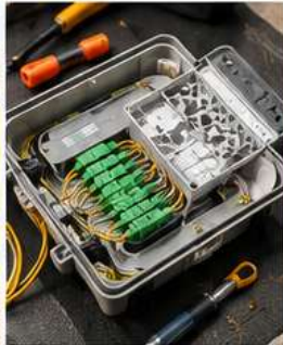
07 FIBER OPTIC INSTALLATION Splicing, termination and testing of fiber optic cables for high speed connectivity.
