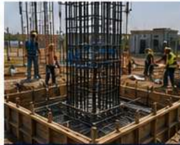
FOUNDATION REINFORCEMENT Reinforcement, formwork and concrete pouring as per structural design.
