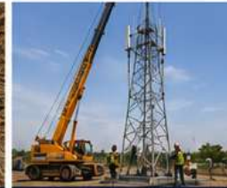
TOWER ERECTION Erection of tower sections using crane and safety equipment.
