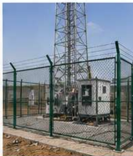
13 FENCING & SITE SECURITY Installation of perimeter fencing, gates and security systems for site protection.
