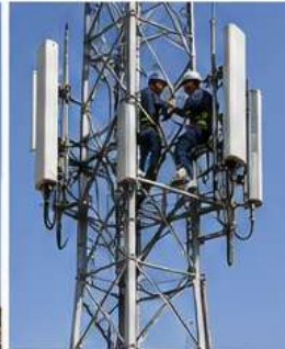
09 ANTENNA INSTALLATION Installation of antennas, RRUs and microwave dishes at required heights.
