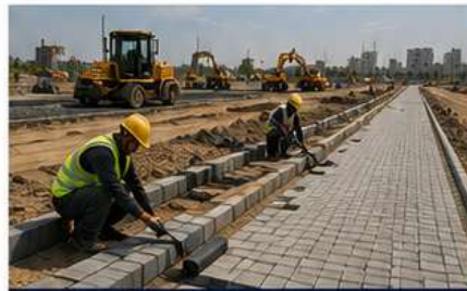
9. PAVING & SITE DEVELOPMENT Interlocking, kerbs, road works and external development for durable finishes.
