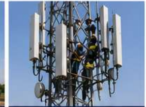
ANTENNA & RRU INSTALLATION Installation of antennas, RRUs and microwave dishes.
