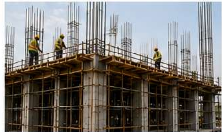
4. FORMWORK & SHUTTERING Installation of formwork systems ensuring strength, safety and accuracy.
