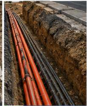
05 DUCTING & CONDUITS Installation of HDPE ducts and conduits for power, telecom and fiber cables.
