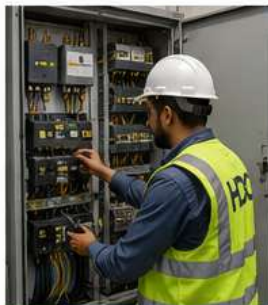
11 ELECTRICAL & POWER SYSTEMS Installation of power distribution, DBs, AC/DC systems and backup power solutions.
