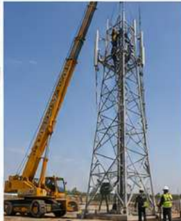
08 TOWER ERECTION Safe erection of telecom towers using cranes and skilled technical team.
