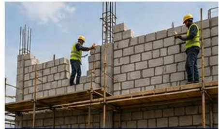
7. MASONRY & BLOCKWORK Brickwork, blockwork and partition walls with neat finishing.
