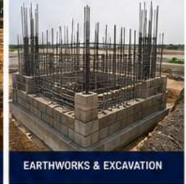
TOWER FOUNDATION WORKS
