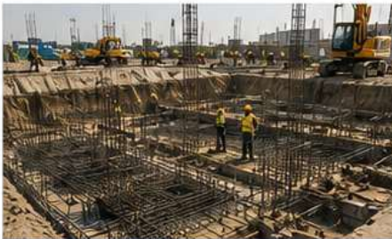
2. FOUNDATION WORKS PCC, footing, raft and pile foundation works with precision.
