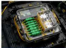
FIBER OPTIC SPLICING Fiber optic splicing, termination and testing for reliable connectivity.
