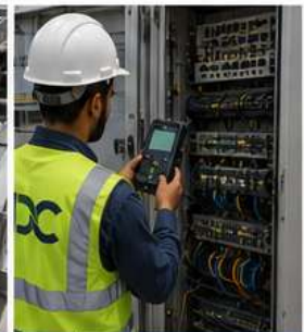
15 TESTING & COMMISSIONING Testing, integration and commissioning to ensure optimal performance.
