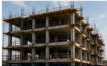
6. STRUCTURAL FRAME WORKS Erection of columns, beams and slabs forming the main structural frame.
