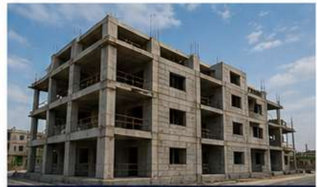
10. COMPLETION & QUALITY CHECK Final inspection, quality assurance and handover with complete documentation.
