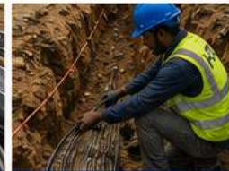
CABLE PULLING & LAYING Pulling and laying of power, telecom and fiber optic cables.
